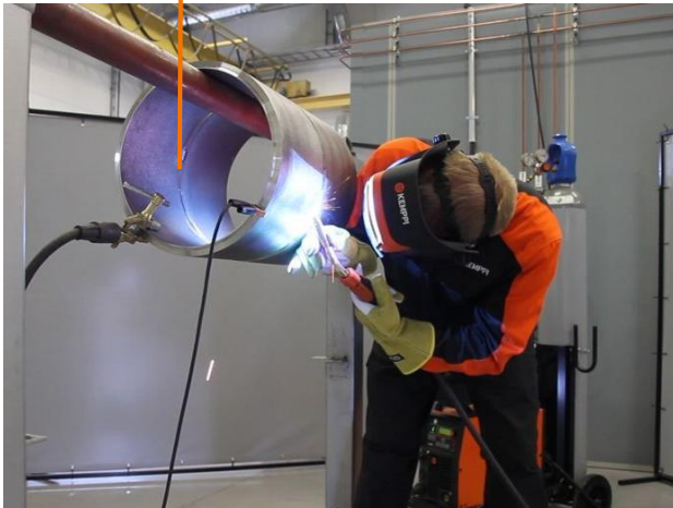
Fig. 8. Fixed pipe welding.
